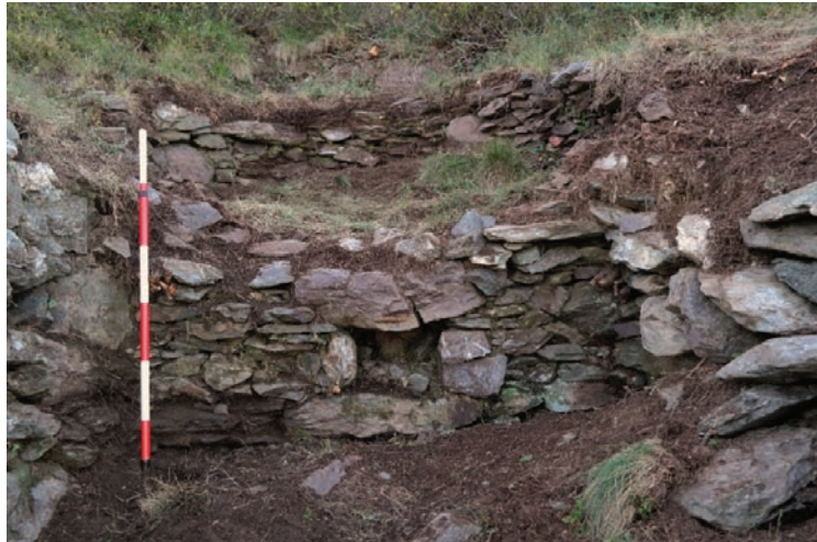
Figure 15. Fusine (SONDRIO), Val Cervia, roasting furnace to the north of the mine. Detail of the façade of the combustion chamber of the furnace with a small opening at the centre for unloading the iron ore.
