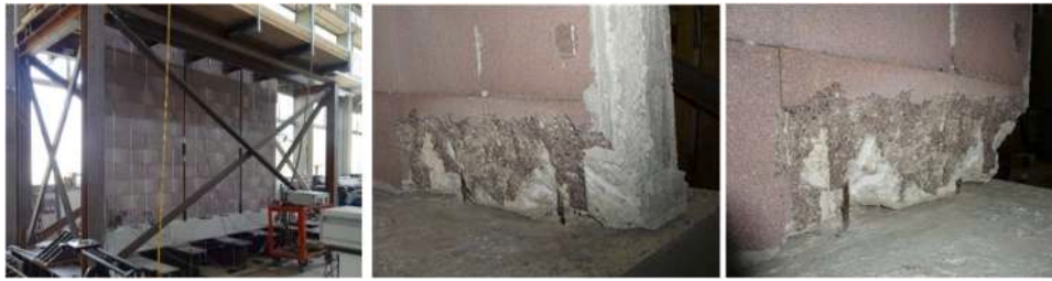
Fig. 13. Tests' execution and damages in correspondence of the connection between the foundation system and the sample.
