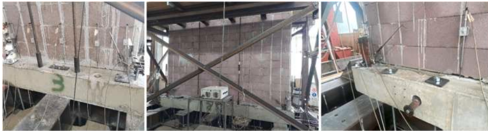
Fig. 15. Cyclic tests' execution and details of damage in correspondence of the RC foundation connections (1:2 and 4:3).
