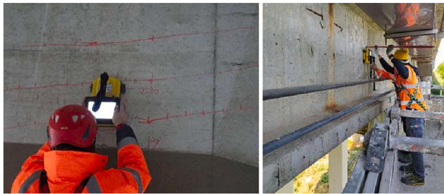
Fig. 7. GPR execution in situ.
