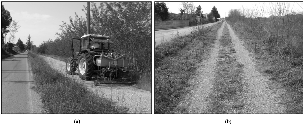
Figure 11. Mounted flaming machine at work (a) and an overview of the gravelled cycleway.
