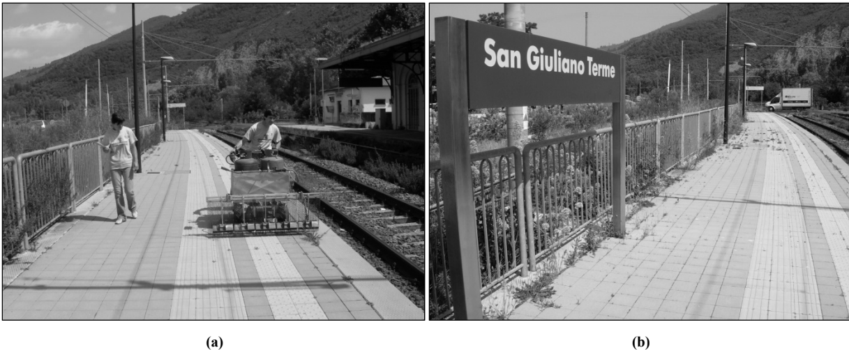
Figure 10. Self-propelled flaming machine at work (a) and the railway station (b).
