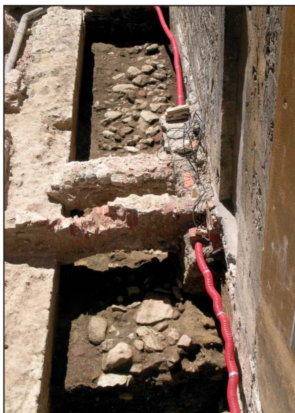
Fig. 3.52 Excavation of via degli Uffizi. The alley (chiasso) between tower houses A and B.
