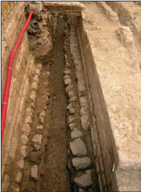
Fig. 3.47 Excavation of via degli Uffizi. The foundations of tower houses A, on the left, and B, on the right.
