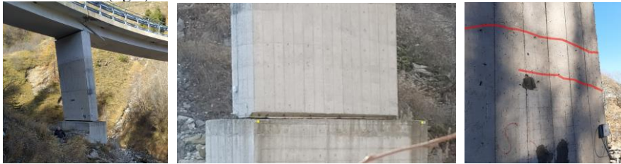
Fig. 2: View of the current configuration of pillar 1.
