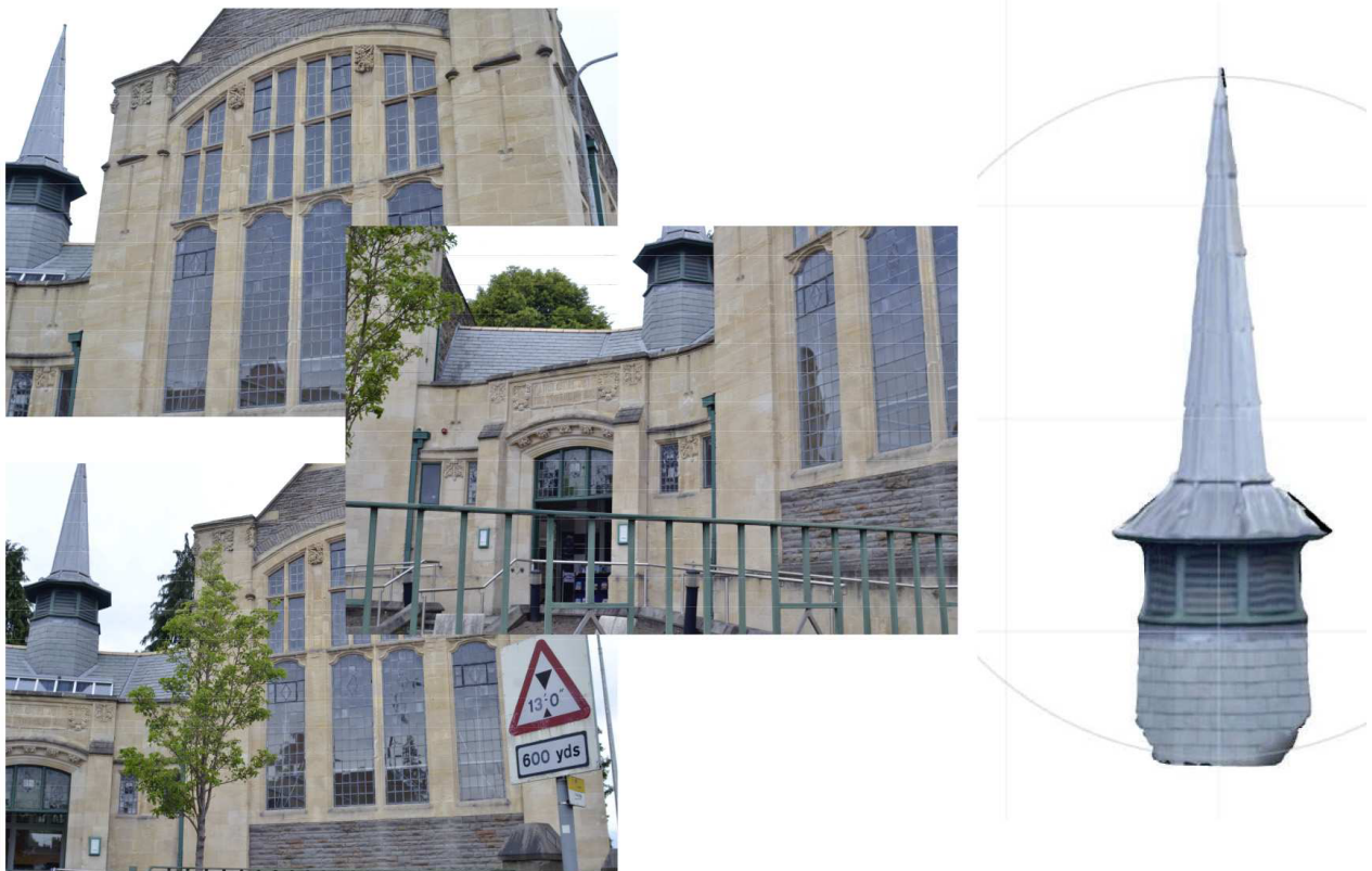
Figure 6. SFM: mesh of the ventilation tower
