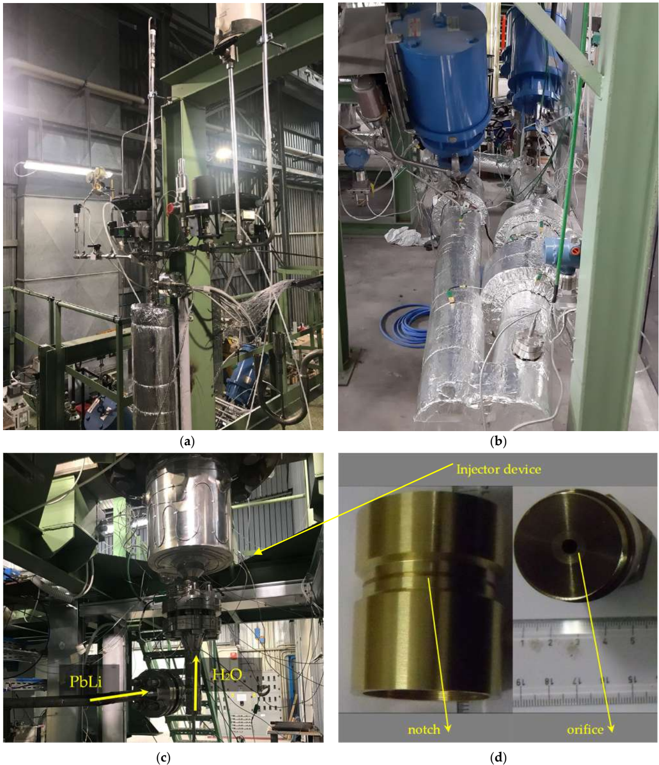
Figure 5. Detail of the injection line and device. (a) Upper part of the water injection line connected to argon gas cylinder; (b) injection line with valves and Coriolis; (c) injection piping and connection to the S1B vessel; (d) injector cover brass cap with specified notch dimensions.
