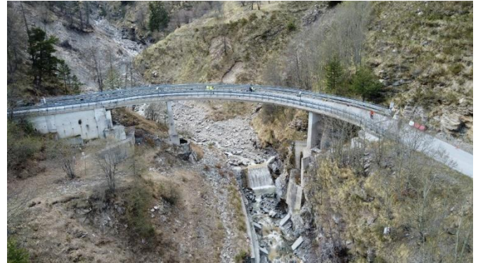
Figure 1 Case study: curved roadway bridge in Italy.
