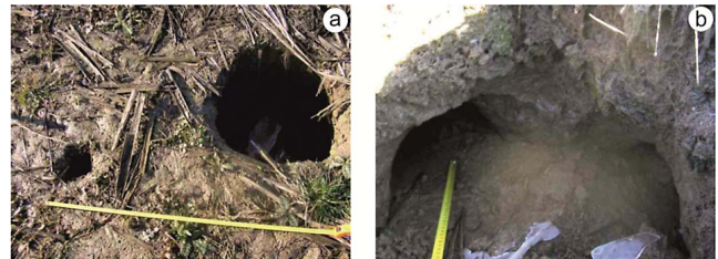
Fig. 8. (a) Vertical conduit (left) and sinkhole-like feature (right); (b) sub-horizontal tunnels departing from the bottom of the cavity.
