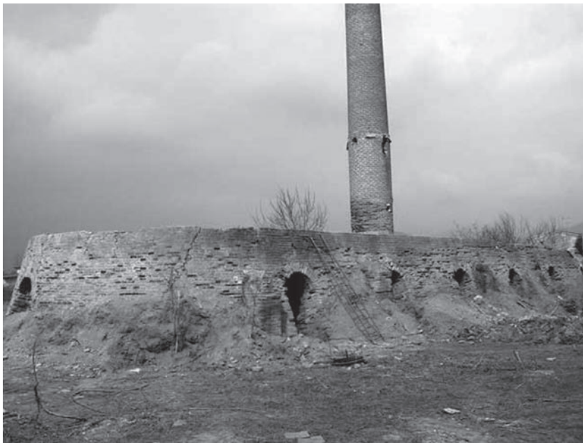
A Hoffmann kiln at San Giuliano Terme (2005, photo by Torti)
