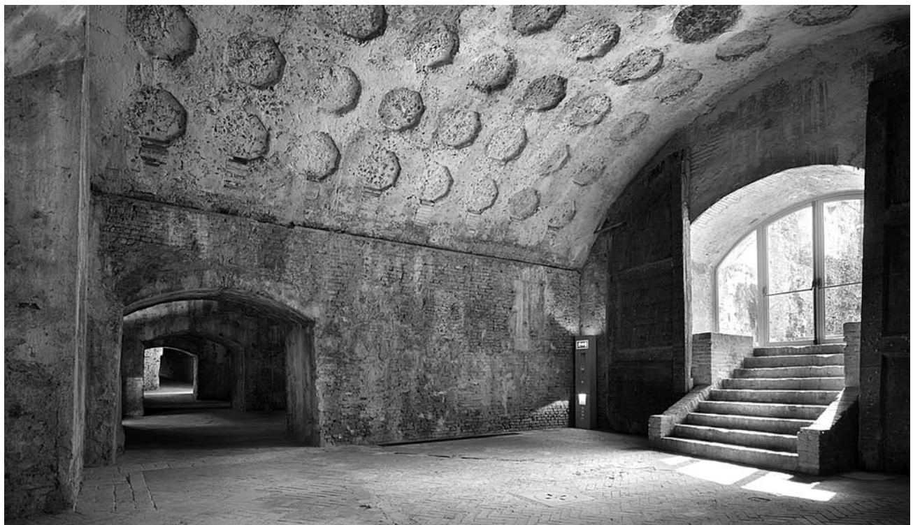
Figure 18 Entrance hall to the underground chambers of the bastion of San Martino, Pisa (photo by Mario Ciampi, with permission of the Comune di Pisa).
