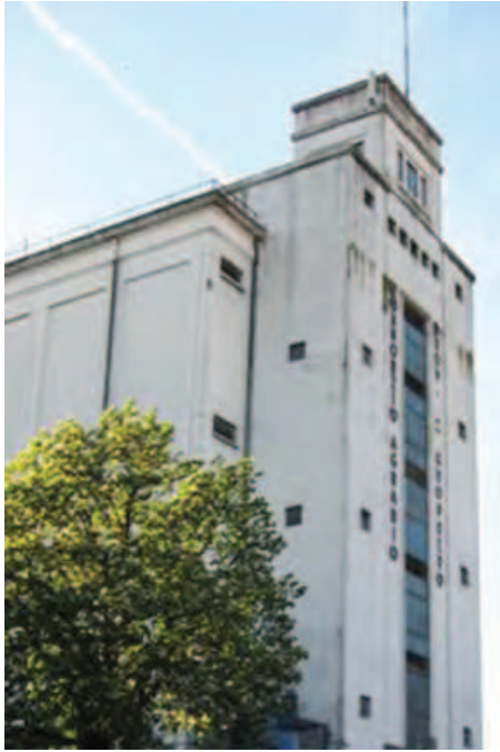
Figure 2 Main façade of the silo
