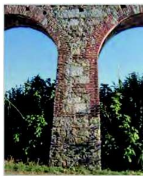
Figure 14 Pillar between arches nr.837 and 838
