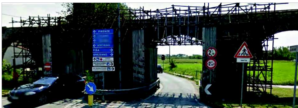
Figure 26 Arches nr. 394 and 395, provisionally supported
