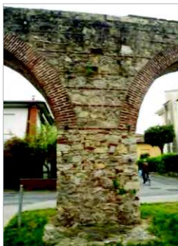
Figure 13 Pillar between arches nr.131 and nr. 132
