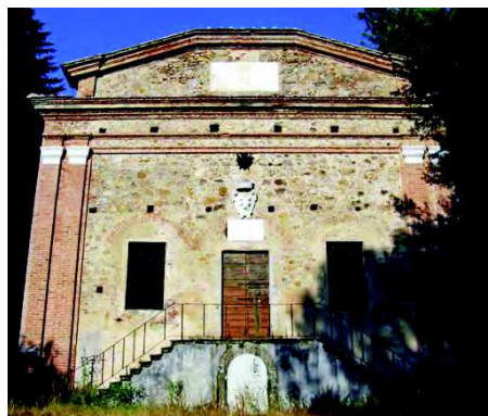
Figure 4 “ Il Cisternone ”, a big cistern for collecting water, in Asciano
