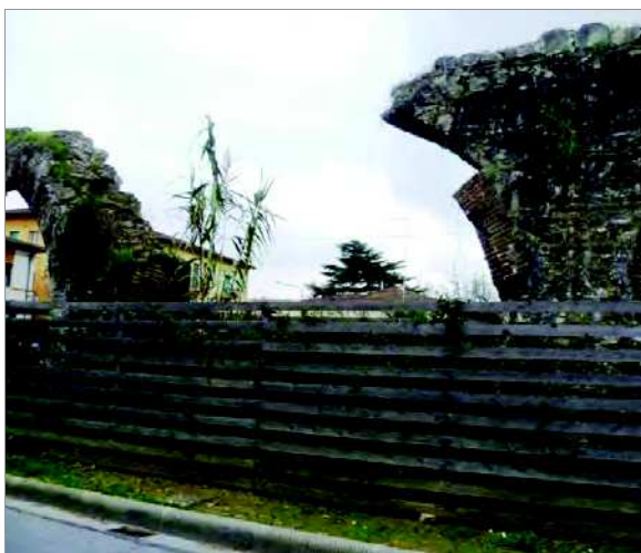
Figure 21 Arch nr. 99, collapsed
