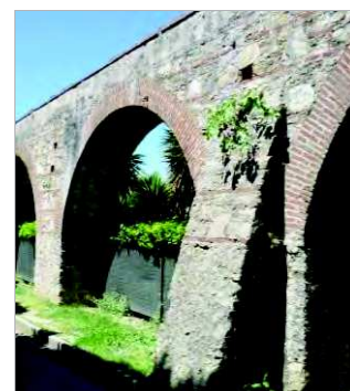
Figure 17 Buttress between arches nr. 199-200
