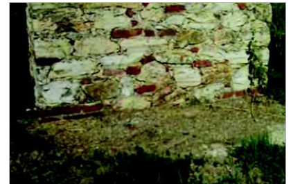
Figure 20 Base under the pillar, between arches n°410-411
