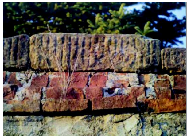
Figure 9 The sheet of stone that covers pipeline
