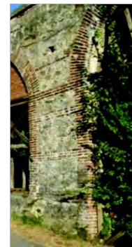
Figure 15 Pillar between arches nr. 815 and nr.816
