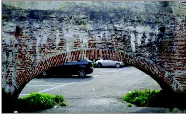
Figure 23 Arch nr. 49, rebuilt in bricks
