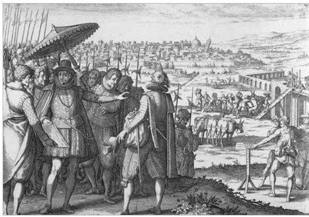
Figure 2 View of the Medicean Aqueduct, in 1600, during the erection
