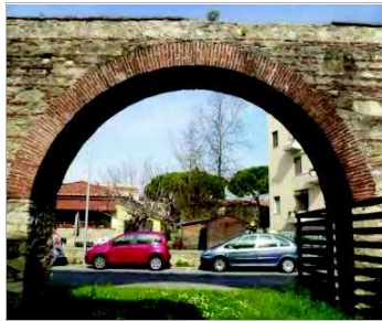
Figure 10 Semi-circular arch (arch nr. 98)
