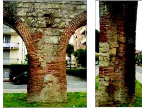
Figure 24 Pillar of arch nr. 130, rebuilt in bricks
