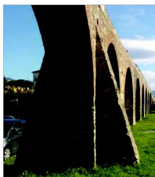
Figure 16 Buttress between arches nr. 89-90
