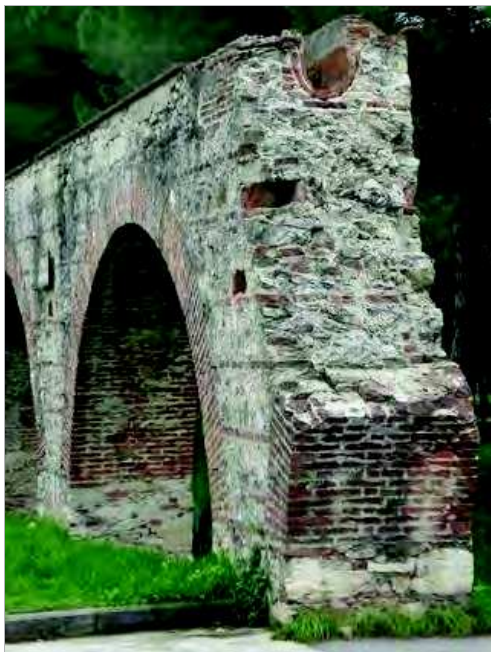
Figure 8 Arch nr. 58, where the core structure and the clay pipeline are visible
