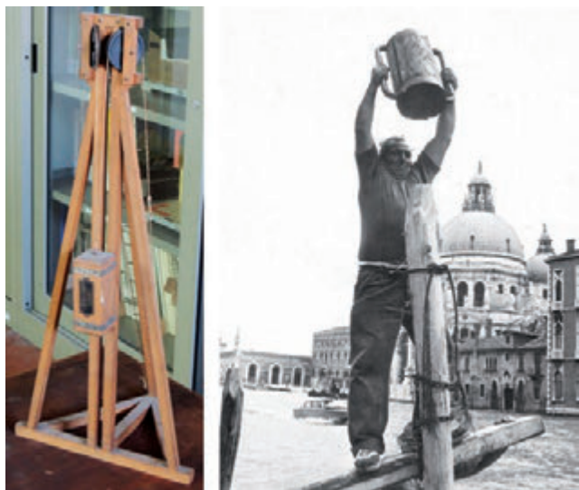
Figure 1. Pile driver model, owned by the GESAAF, and a present-day hand operated pile driver in Venice.
