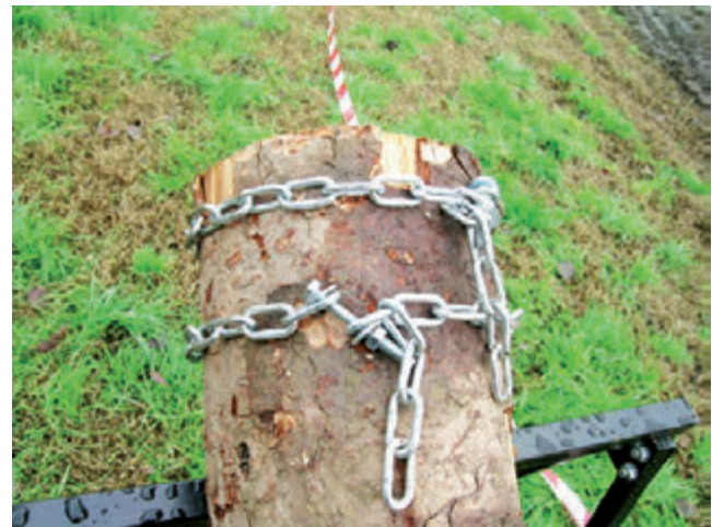
Figure 4. Pile head frettage.
