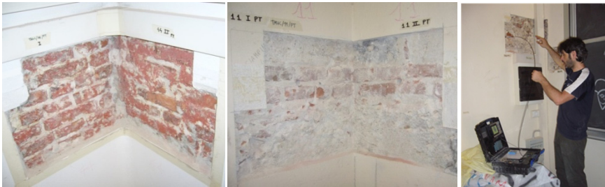
Figure 6: Endoscopic investigations on masonry walls (Palazzo La Sapienza).
