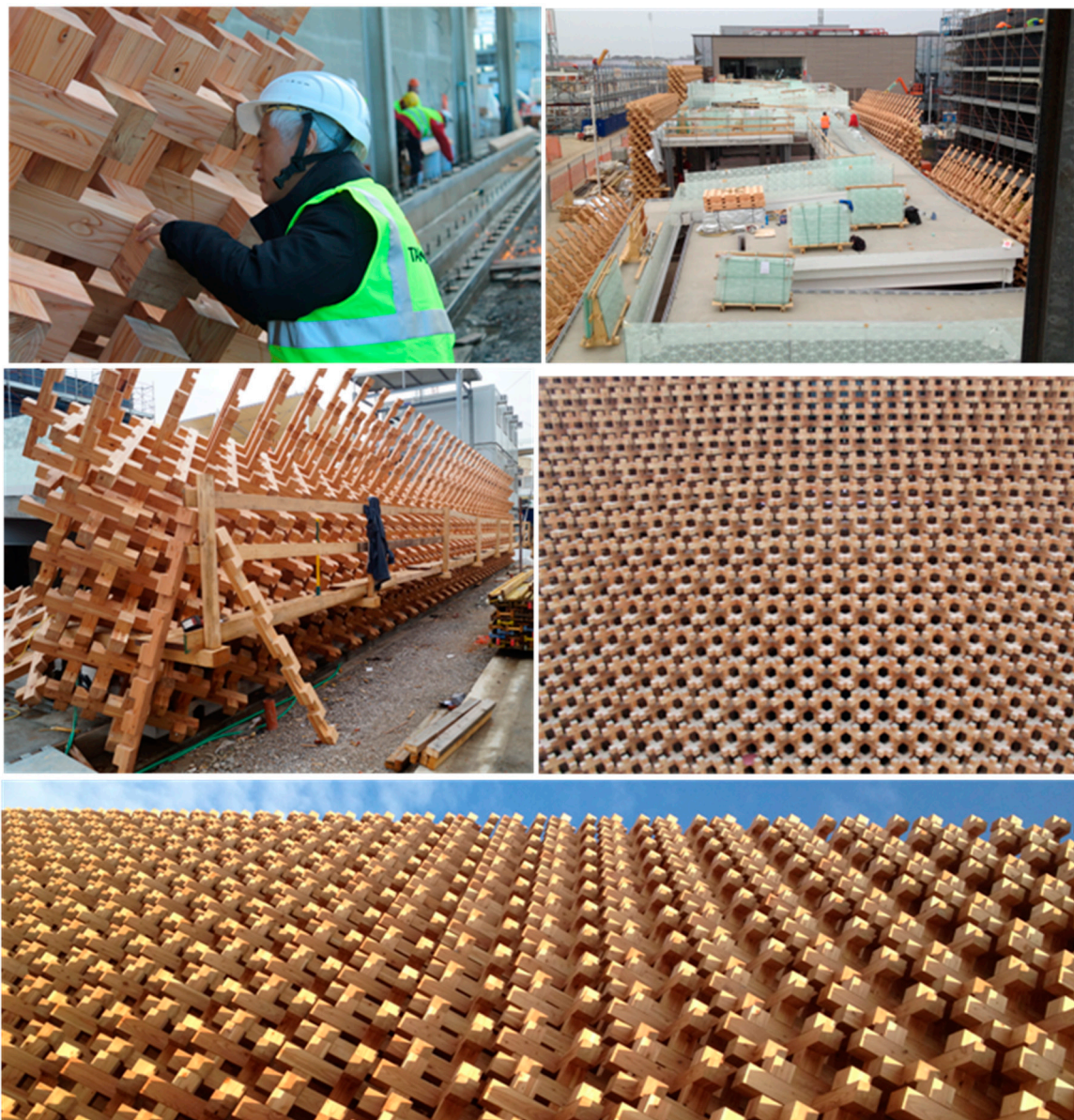
Figure 9. Views of the working phases (source: Galloppini Legnami).
