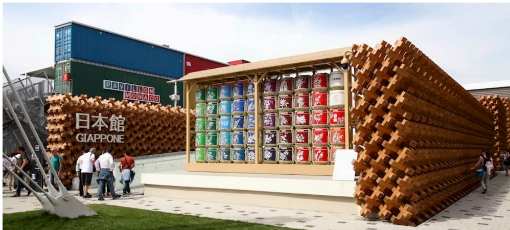
Figure 10. The Japan Pavilion at Expo 2015 in Milan (source: official web site of Expo 2015).
