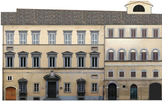
Fig. 2. The facade on via San Martino.
