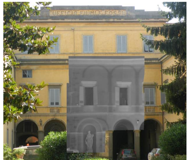
Fig. 6. Superposition of IR and visible images of the facade fronting the Arno river.
