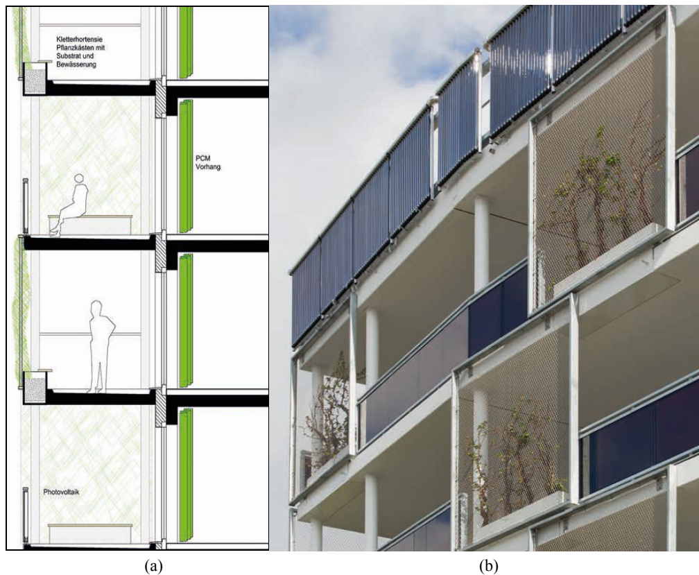
Fig. 6 Residences in Hamburg: (a) section; (b) perspective. PCM integration into façade and PV-vacuum tube collectors on the parapet wall.
