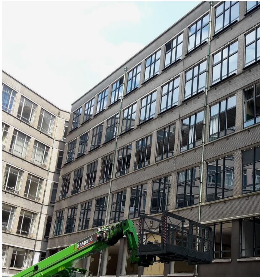
Fig. 9 Haute Ecôle, Belgium. Retrofitting façade with replacement windows. Block No. 6, patio, perspective. Source: Ref. [18].
