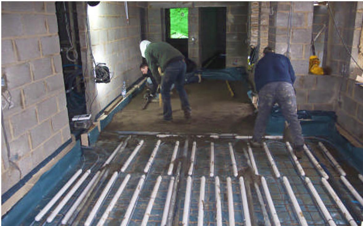
Fig. 5 Underfloor energy storage with PCM materials.
