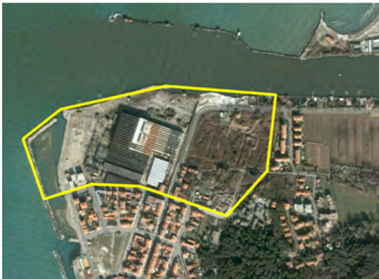
Fig. 1. Area intended for marina construction, before work – October 2007 (image from Google Earth)
