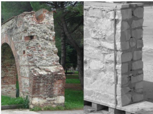
Figure 2: The masonry of the Medicean Aqueduct of Pisa, Italy (left) and a sample of the masonry wall tested in Magenes et al. [13] (right).
