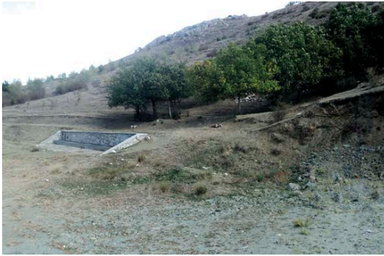
Figure 4. The spring at the base of Kaletepe.
