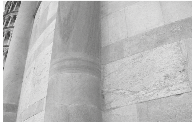
Figure 2 - Detail of the wall of the first storey, showing Monte Pisano marble, Carrara marble and Proconnesian marble.
