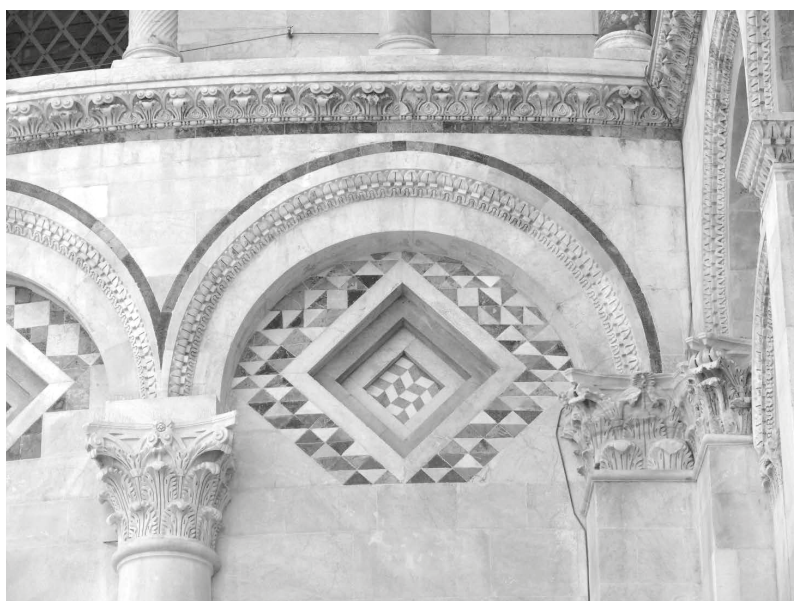
Figure 5 - Detail of the ornamental area of the first storey.
