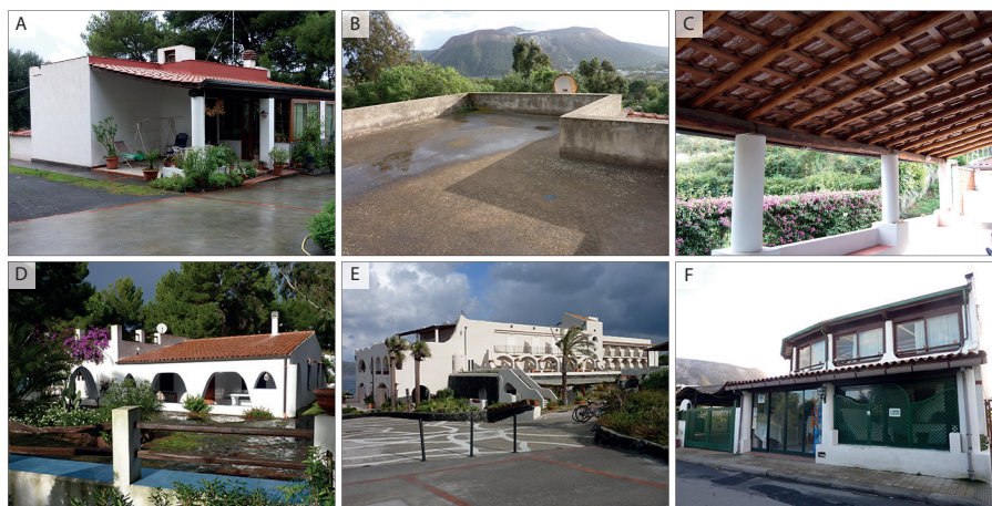
Fig. 6 Typical buildings on the island of Vulcano. A–C Most representative type of residential building, typically single-storey with a concrete flat roof ( B ) and a timber front porch ( C ). D residential building with a roof made of a timber structure and tiles. E Typical one to three storeys hotel complex and F typical commercial arcade in the Porto area. Following the classification of (Spence et al, 2005), buildings shown in A, B, C and E are classified as medium strong (MS) or strong (ST), and buildings D and F as weak (WE) or medium weak (MW).
