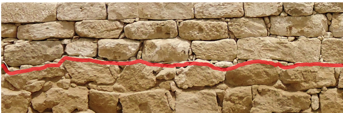
151 Figure 3. Piece-by-piece reconstruction phases: (upper) works in progress, (lower) wall textures with 152 indication of the geotextile (original-under the line, reconstructed-over the line). 153
