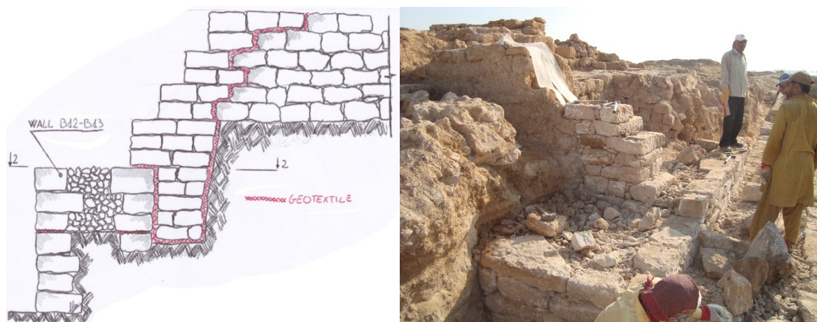
Figure 5 - New buttresses to sustain the building behind city walls
