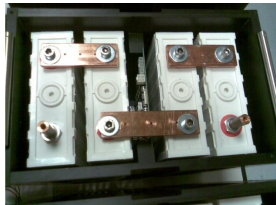
Figure 19: Inside view of the 100 Ah module
