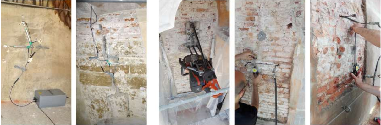
c) installation of the monitoring system.
