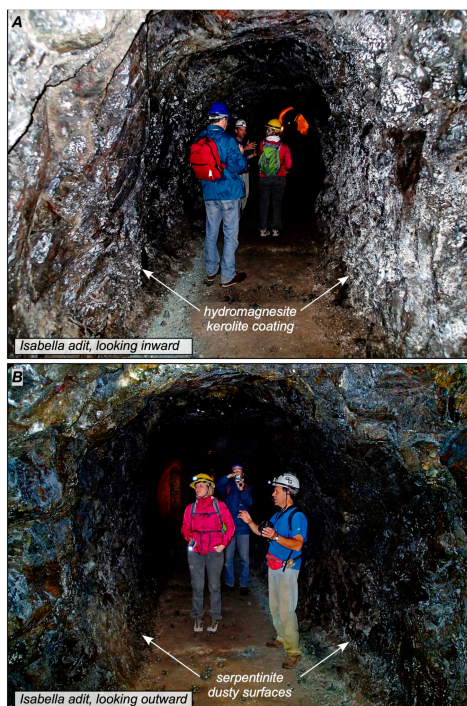
Figure 2. Isabella adit of the Montecastelli mine. (A) View of the adit looking inward where the white coating of hydromagnesite + kerolite and aragonite is visible and (B) view from the adit looking outward where the white coating is not visible.
