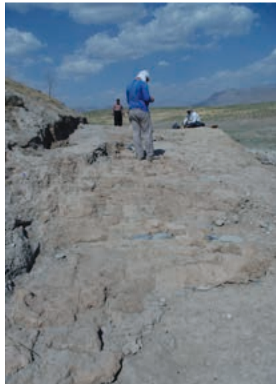
Fig. 12. Lower north slope of Main Hill (view towards west) showing large brick wall (Level IX), founded directly on the natural hill, but “anchored” with a shallow layer of sherds and pebbles.
