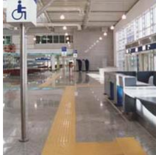
Figure 12. Loges-Apice path installed in a public building
