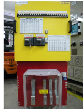
Fig. 11. Active load used during the measurement campaign to modify the operating conditions of each power transformer under test.
