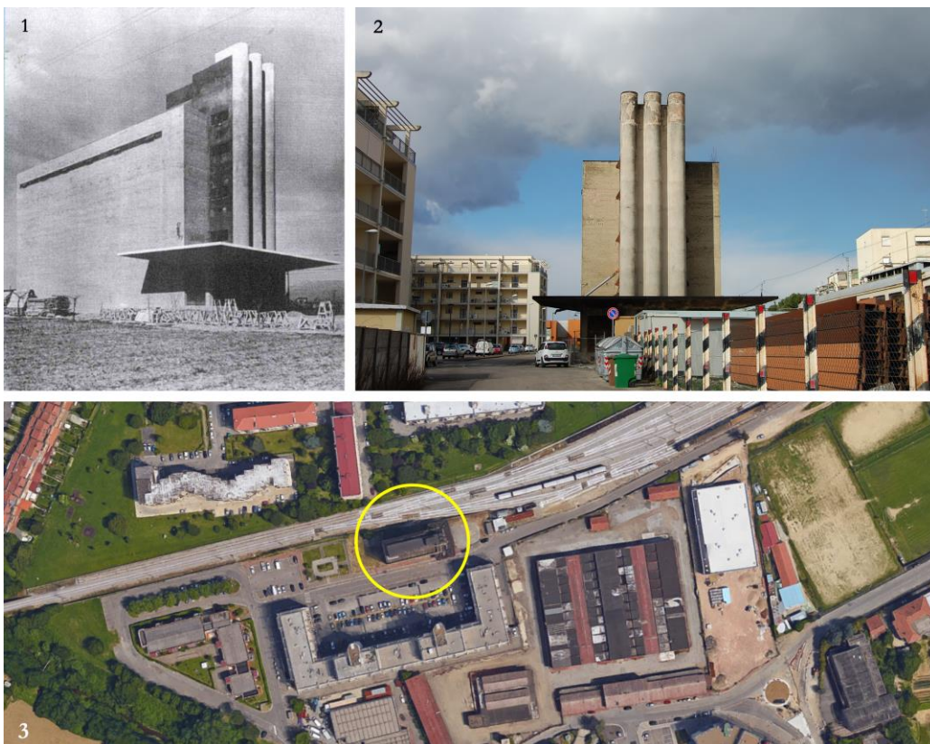
Figure 3. The grain silo of Arezzo (Italy). Historical (1) [29] and current (2) pictures of the building. Location and site plan (3).
