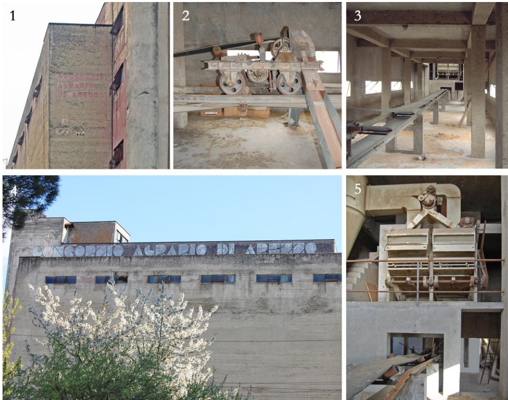
Figure 5. The grain silo of Arezzo (Italy). Architectural and technological elements of the building. 1) Historical writing on the main façade; 2) Horizontal conveyor on the terrace floor; 3) Terrace floor; 4) Historical writing on the side façade next to the railway station; 5) Machineries on the terrace floor.
