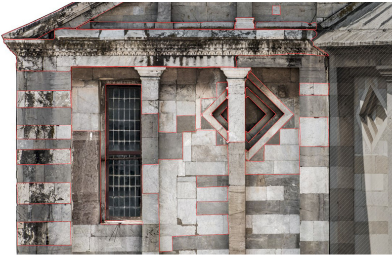
Figure 8. Example of annotations of the material ‘white marble’, performed via McNeel Rhinoceros.
