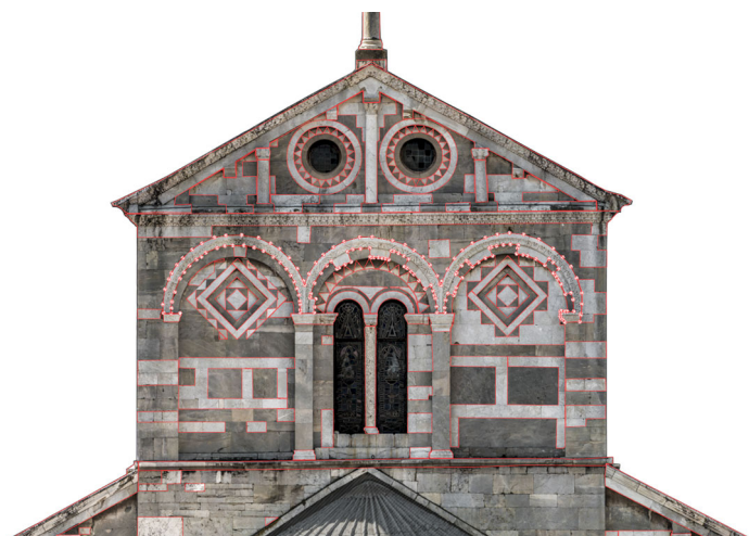
Figure 9. Example of annotations of the material ‘white marble’ in the upper part of the transept, performed via McNeel Rhinoceros.
