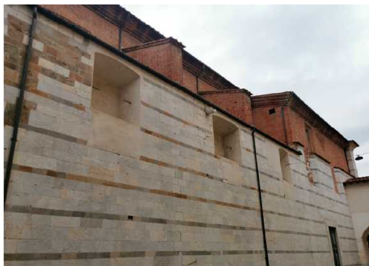
Figure 13. The south wall of St. Nicola Church.
