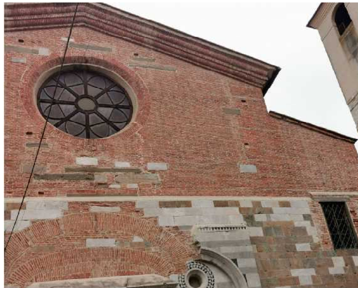
Figure 26. The actual aspect of the main façade—detail (June 2021).
