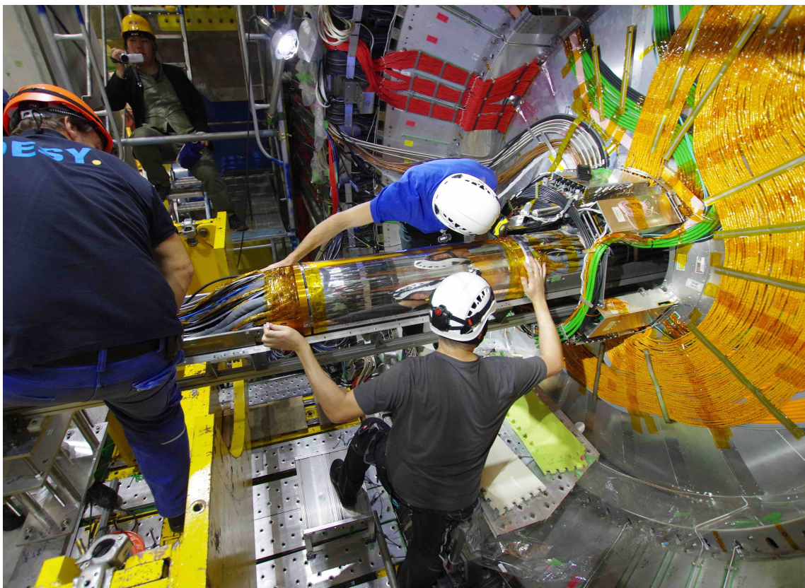
Figure 96. Photo taken during the VXD installation in the Belle II detector: installation of the VXD in the Belle II detector. The slide guide installed in the Belle II detector using the slide guide installed in the forward part of Belle II.
